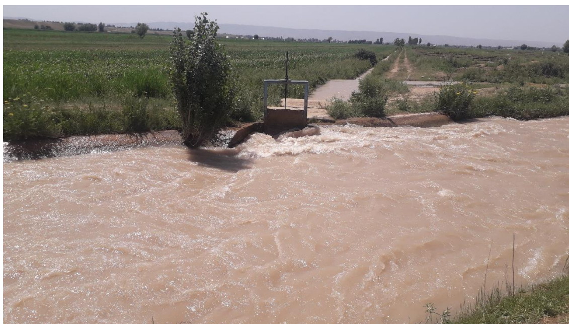
Figure 6. Water outlet on Levaya-Vetka canal, Kara-Unkur-Sai river system, September 2021
