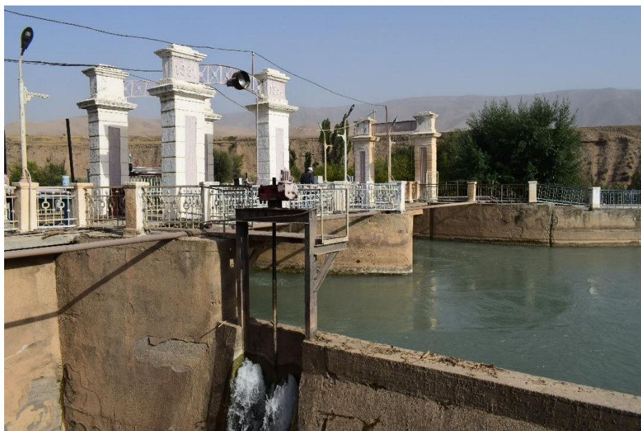
Figure 5. Headwater intake structure on Otuz-Adyr canal, Khurshab-Sai river system, September 2021
