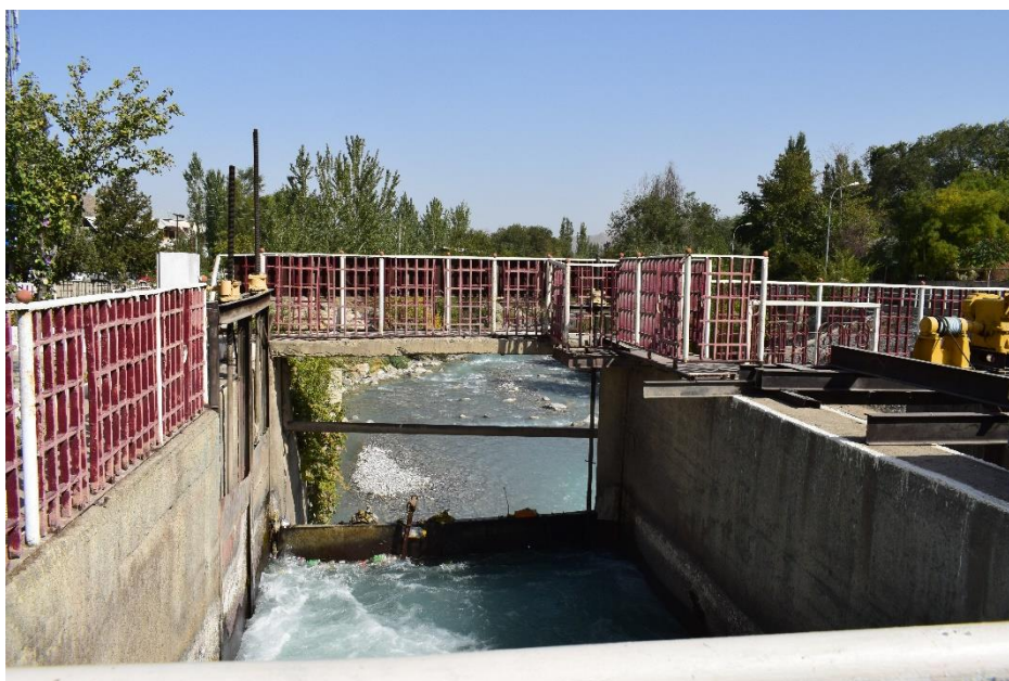
Figure 4. Headwater intake structure on Shakhimardan river, September 2021
