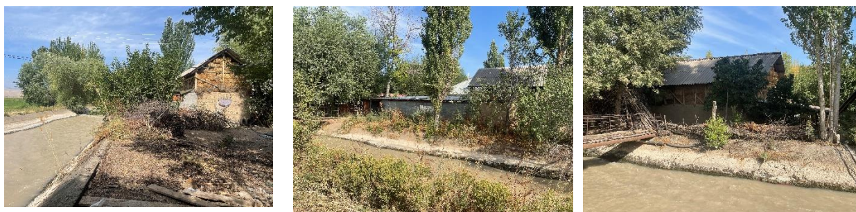
Image 2. Buildings near MC Levaya Vetka from PK39+00 to PK50+00.
