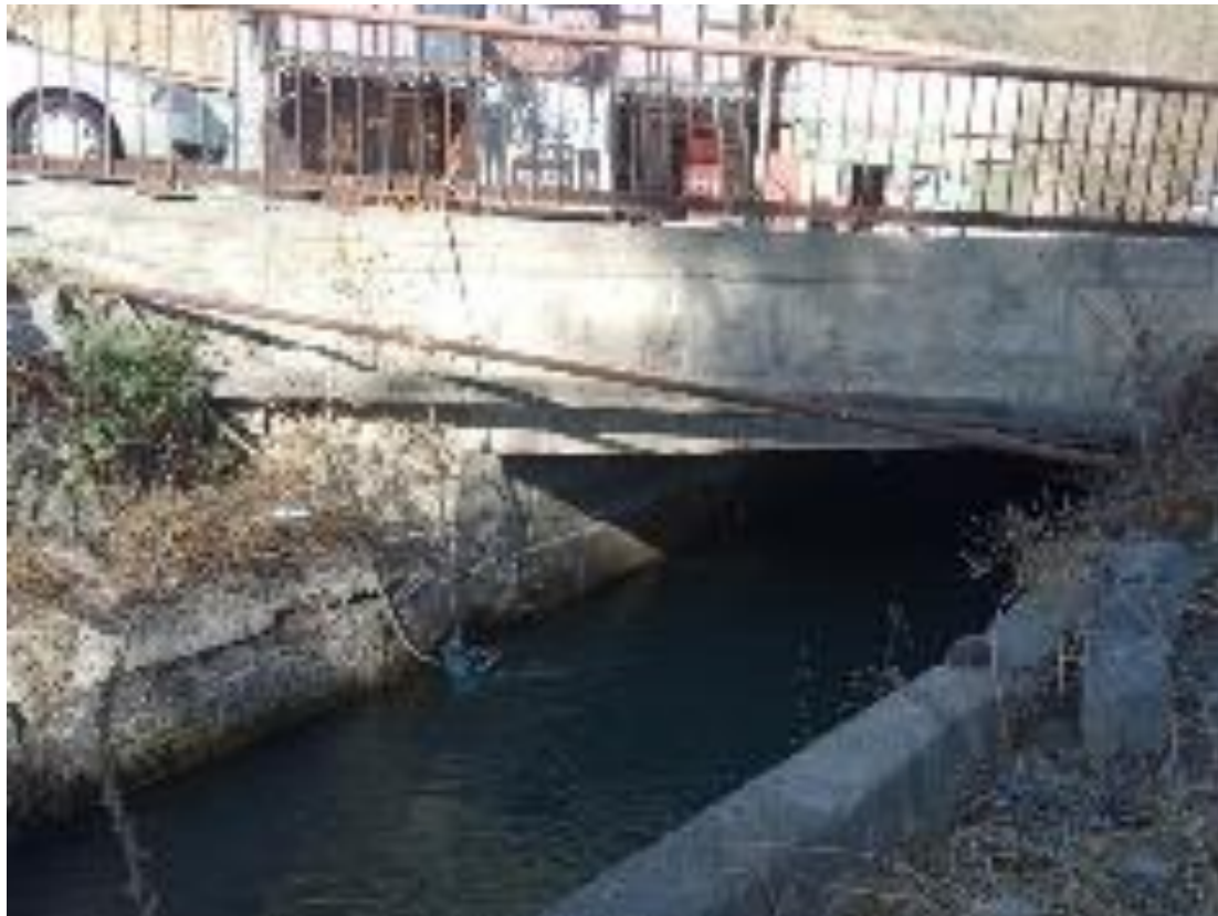
Image 9. Road bridge on PC18+12
