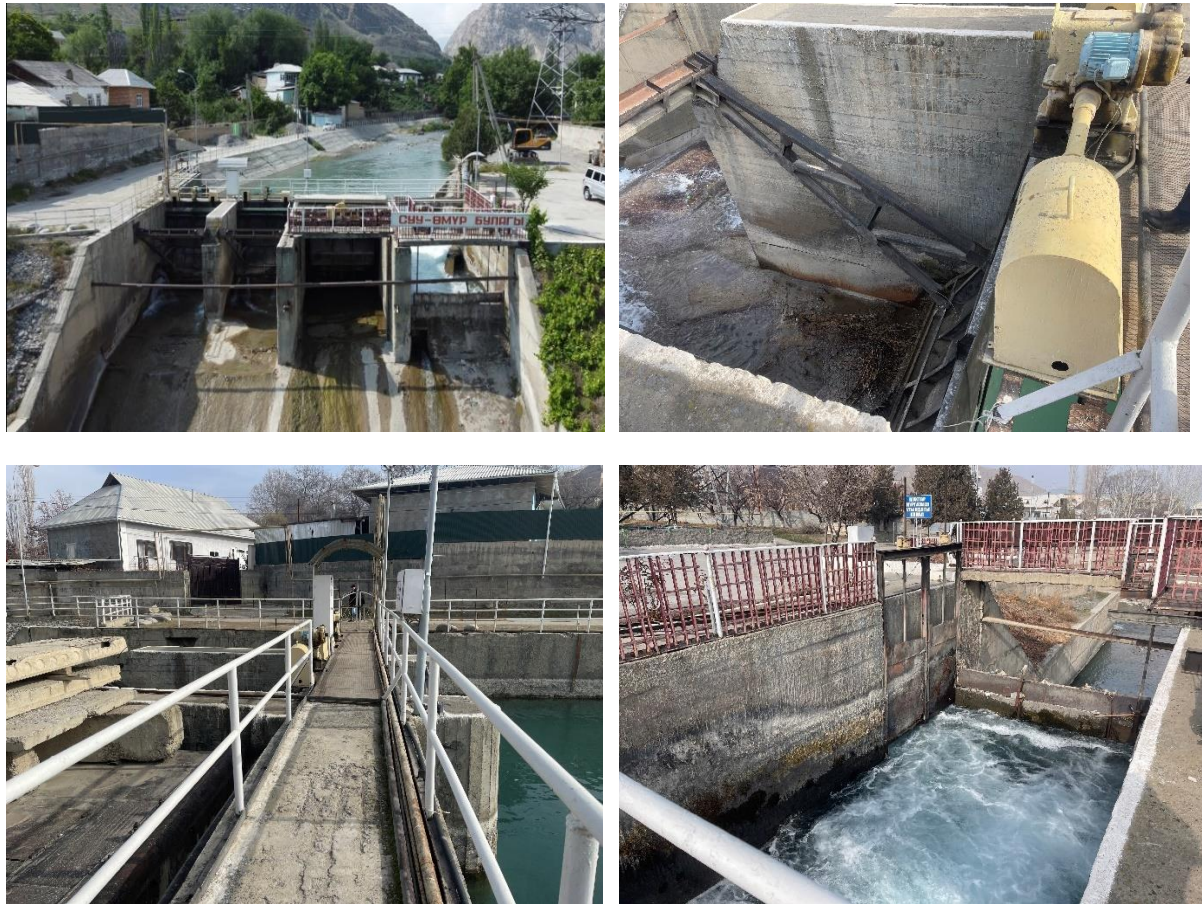
Image 5. Head water intake structure (HWS)
