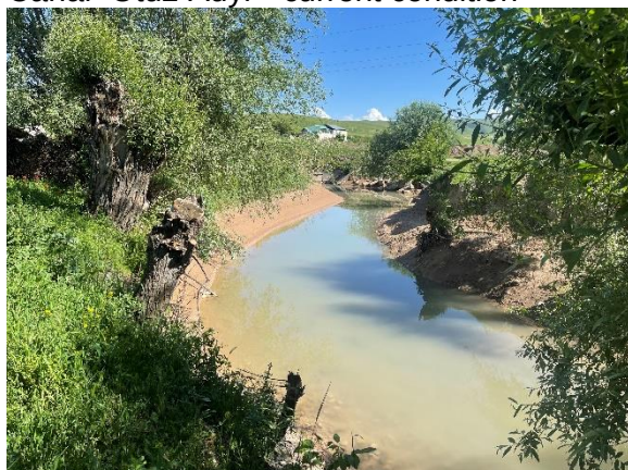
Canal “Otuz-Adyr” current condition
