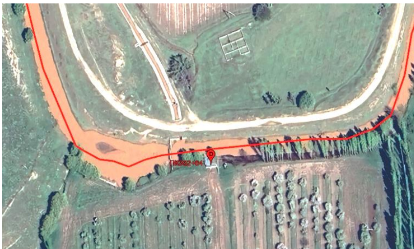
Image 7. Pumping unit shed PK332+64 on the “Otuz-Adyr” canal
